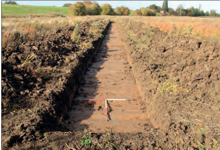
Figure 76: Trench 1046 viewed from the east, scales: 1 m
